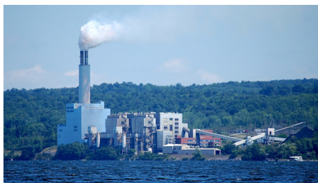
AES' Cayuga plant
